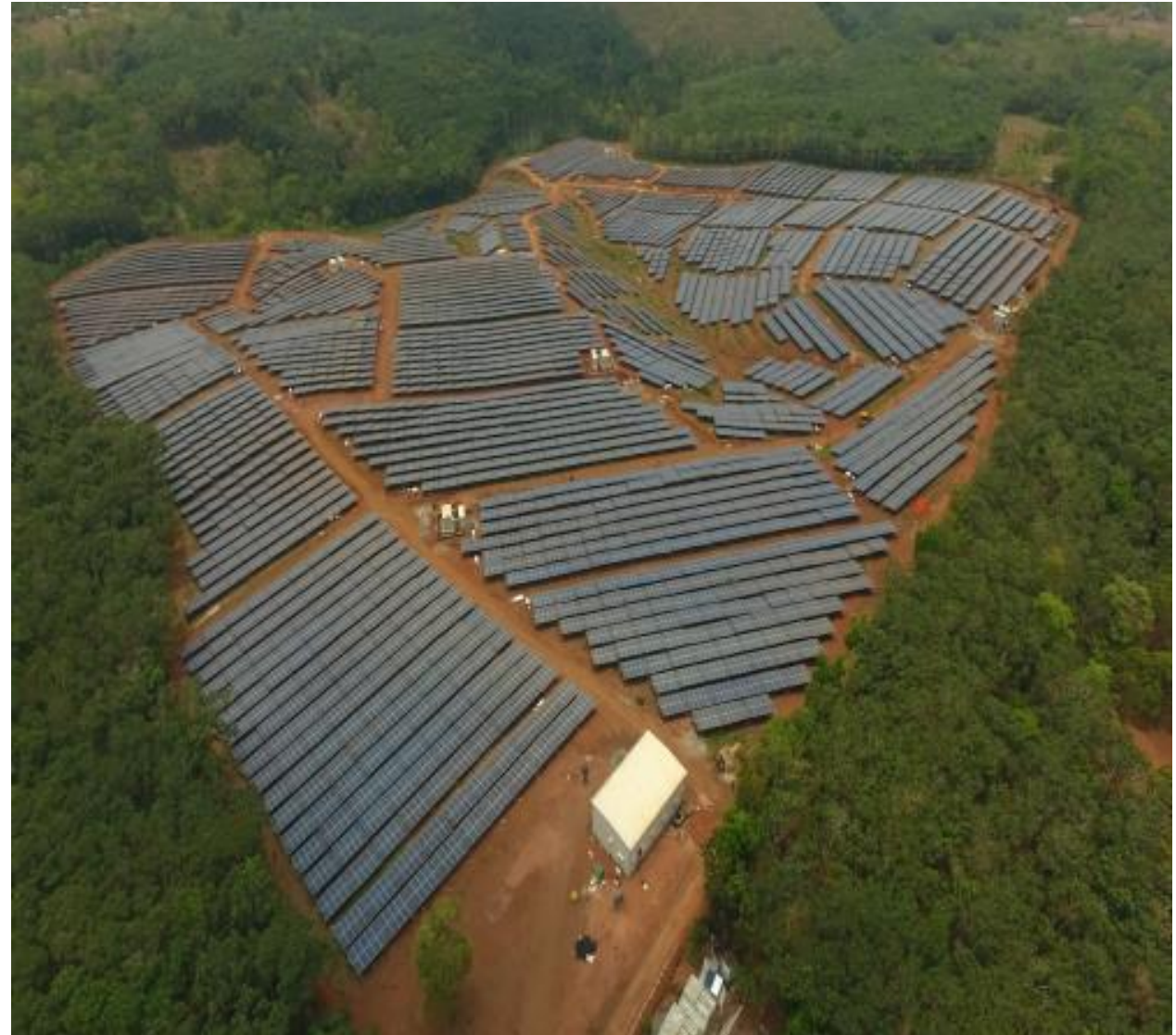
Project Site - After
