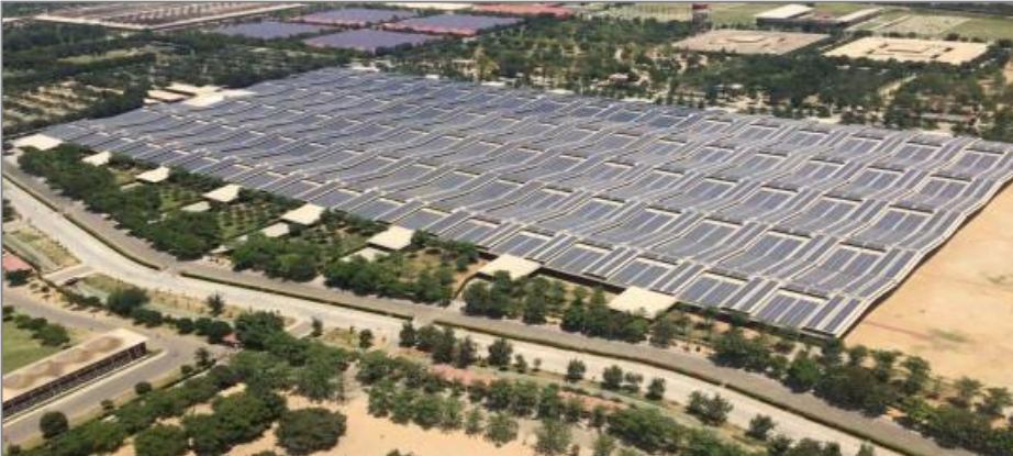
World's largest 16MW Rooftop Solar Plant at R.S.S.B Educational & Environmental Society
